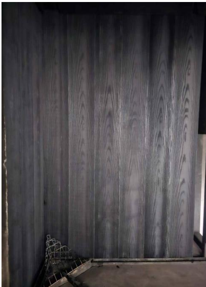
Before test (Long wing)
